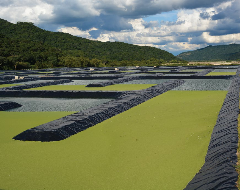
Figure 4.23 Commercial-scale duckweed wastewater treatment project between MamaGrande, a social biotechnology company, and Aguas Del Norte. Salta, Argentina. © 2015 Ryan Gutierrez.
